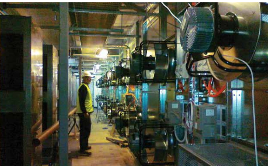
Above: Inside the purpose built containment area that houses the high volume modules (at left) and the fan wall (at right).
